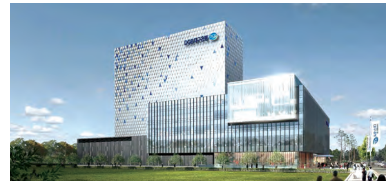
Daegu Bank (DGB) Data Center (PreCon)
